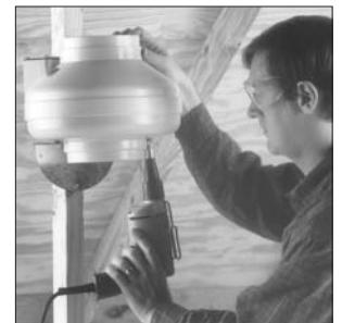
Attach Fan to Mounting Bracket using screws provided.
