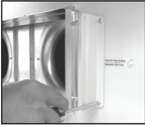
Figure 1 Bracket "B" Installed Support «B» installé
