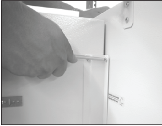
Figure 5 Bracket "B" tightened Support «B» serré
