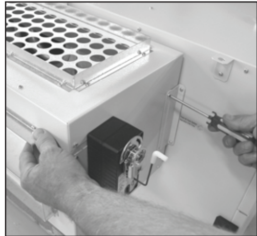
Figure 4 BPM Fastening Fixation du BPM
